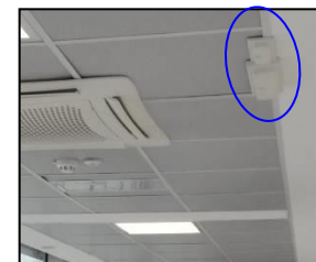
Ceiling-mounted Wi-Fi AP
